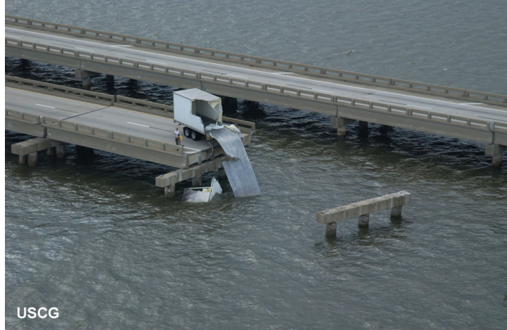
Figure 1.2 Collapse due to huge loading on the partially drifted deck after extreme event.
